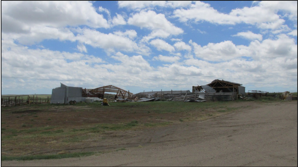
Figure 4.11.4 – June 22, 2016, Severe Storm Damage in Logan County, North Dakota
