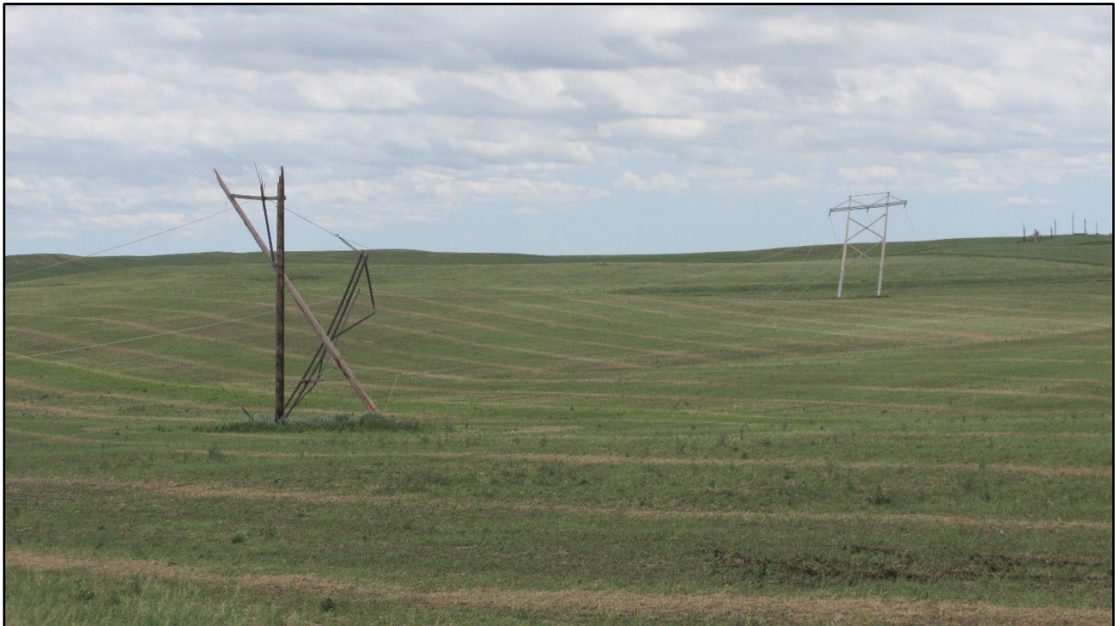
Figure 4.11.2 – June 22, 2016, Severe Storm Damage in Logan County, North Dakota
